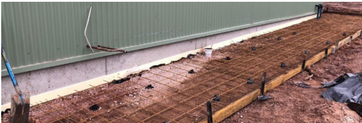
FIGURE 6.5 A GREENZONE® EFTS used as a barrier between the external perimeter of the building and a ramped path/access way.
