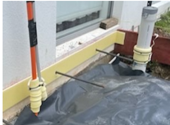
FIGURE 8.6 D GREENZONE® EFTS wrapped 2 conduits; GREENZONE® STS applied to 100mm plumbing pipe; GREENZONE® EFTS to cold joint installation. Dowels inserted through the product.
