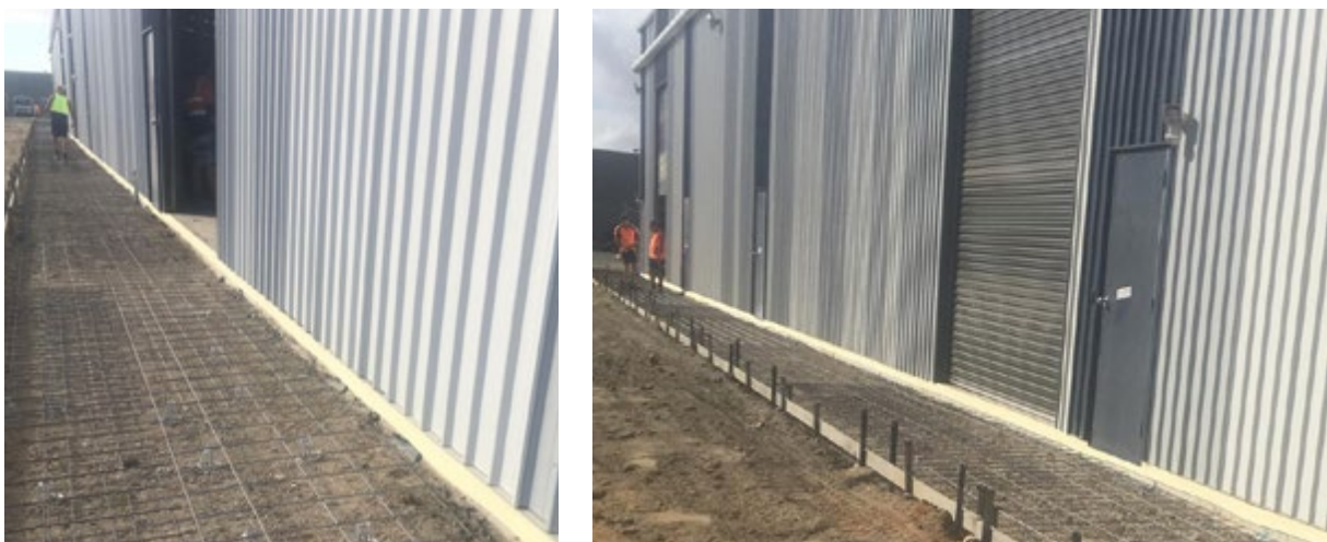
FIGURE 6.5 B GREENZONE® EFTS used as a barrier between the building and an external pathway and across doorways/openings into the building.
