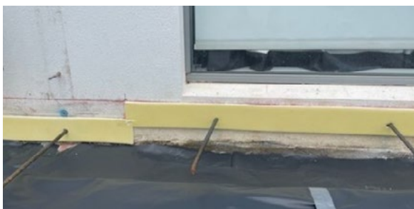
FIGURE 9.6 C Examples of dowels inserted to cold joint installation of GREENZONE® EFTS.
