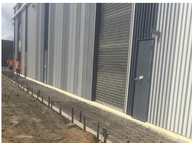
FIGURE 6.5 B GREENZONE® EFTS used as a barrier between the building and an external pathway and across doorways/openings into the building.
