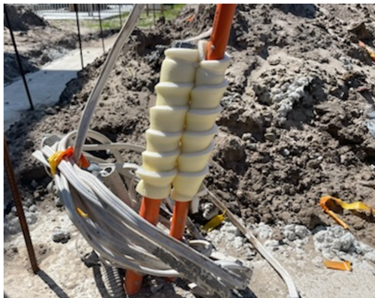
FIGURE 8.6 B GREENZONE® EFTS wrapped to a cluster of 2 conduits.
