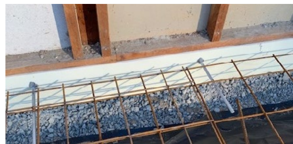
FIGURE 9.6 C Examples of dowels inserted to cold joint installation of GREENZONE® EFTS.
