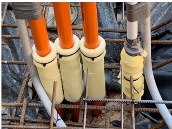
FIGURE 8.6 C GREENZONE® STS applied to 3 orange conduits; GREENZONE® EFTS applied to 1 conduit. Note - 2 grey conduits not treated as they are cast into the slab.
