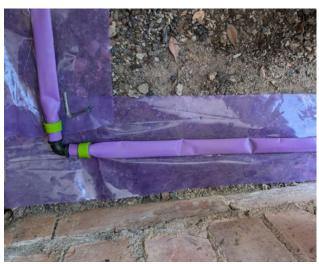
GREENZONE® original Altis Reticulation System protects against the infestation by subterranean termites and is designed to effectively treat the area under concrete slabs, subfloor areas and around external perimeters of structures, preventing termites entering from the outside of a building.
