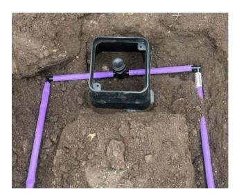
GREENZONE® new Altis Pro Reticulation System protects against the infestation by subterranean termites and is designed to effectively treat the area under concrete slabs, subfloor areas and around external perimeters of structures, preventing termites entering from the outside of a building.
